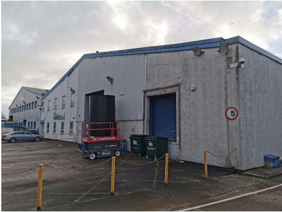
1. Overview of roller shutter entrances to Unit 2a.
