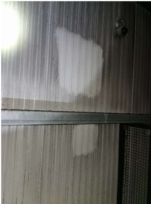
24. Cleaning test panels in Unit 2a.
